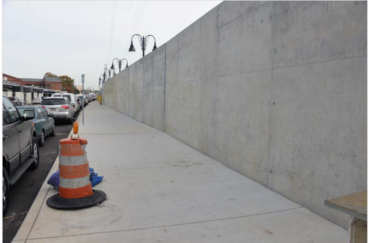
Floodwall at Dumaine Street: Under construction (left) and completed (above)
