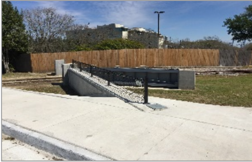
Floodgate at Audubon
