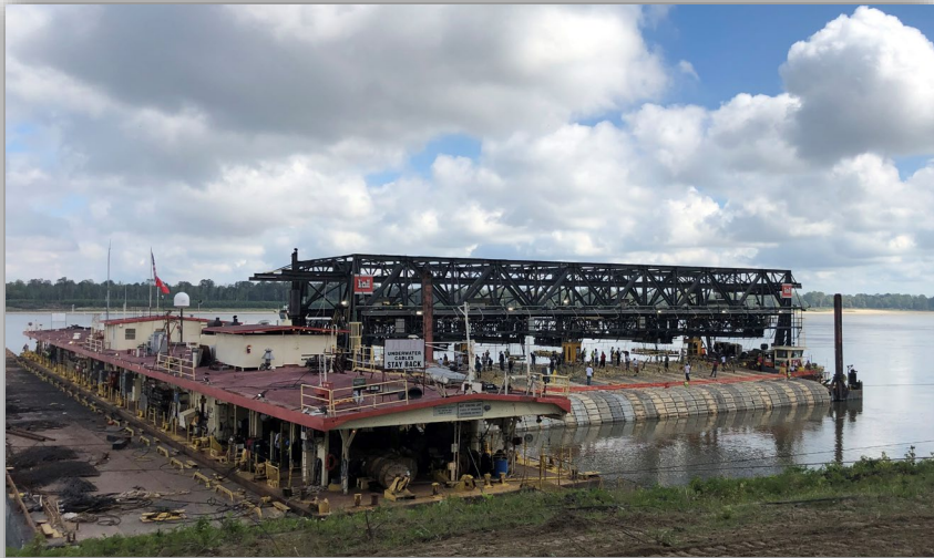
MSU performing flood repairs at Milliken Bend Revetment, Madison Parish, October 2021
