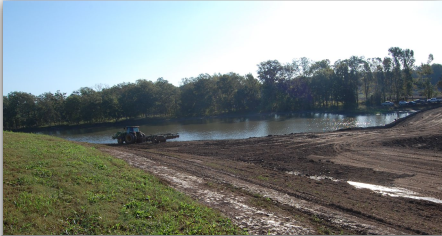
Preparing levee base for lift, MRL Item 401-R, Tensas Parish, October 2021
