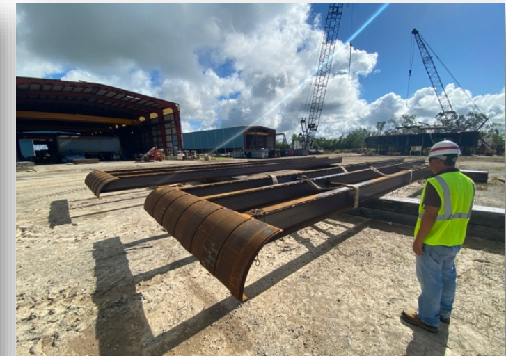
ARMOR 1 construction at Thoma-Sea Shipyard, Houma, LA
