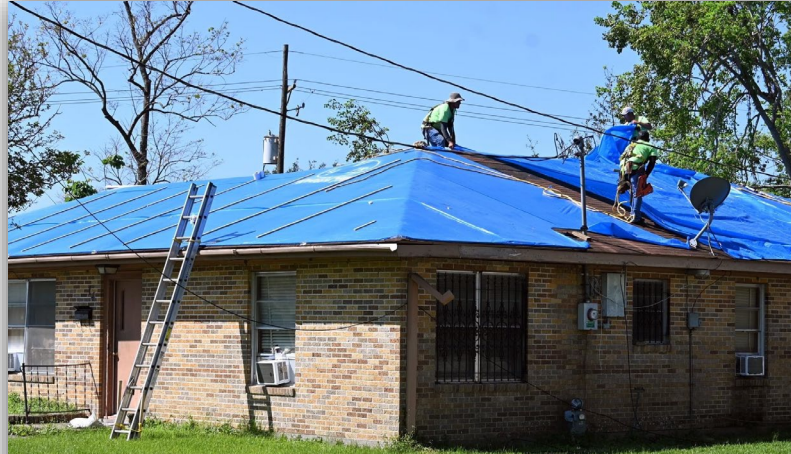
MVK team members donate their time and expertise to the Hurricane Ida Operation Blue Roof Effort in Louisiana, Sept. – Oct. 2021
