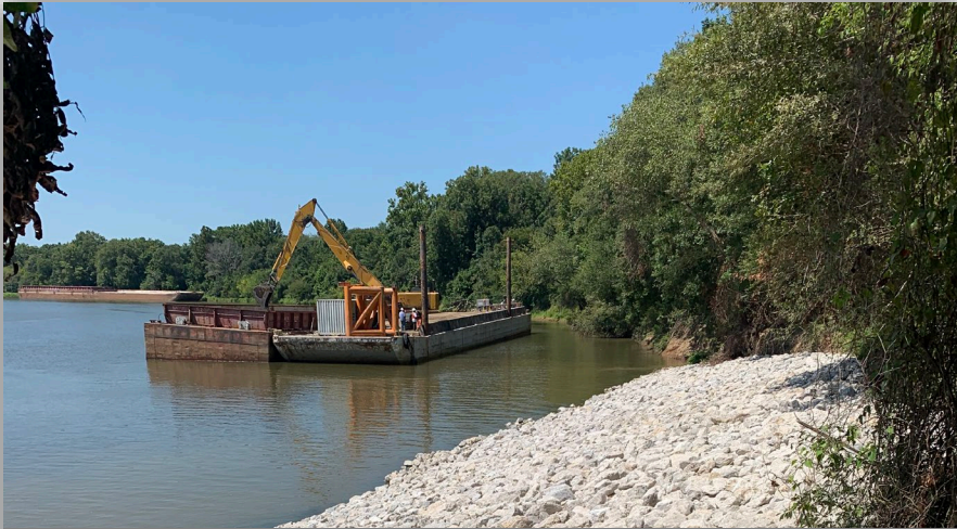
2016 Project, Construction Phase
