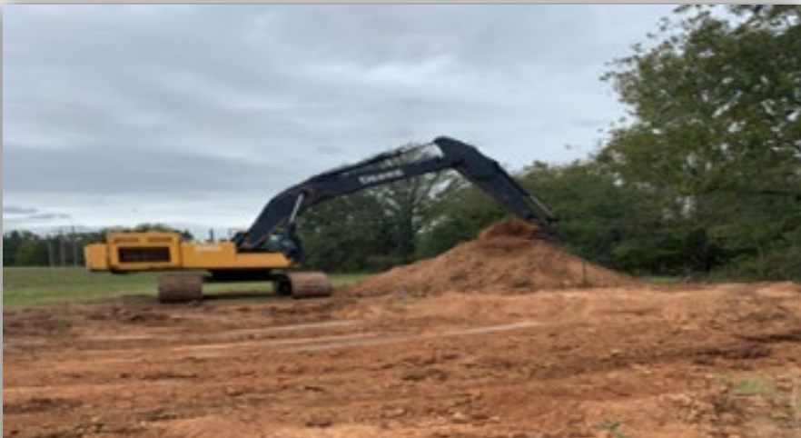
2016 Project, Digging to setup the levee tiebacks
