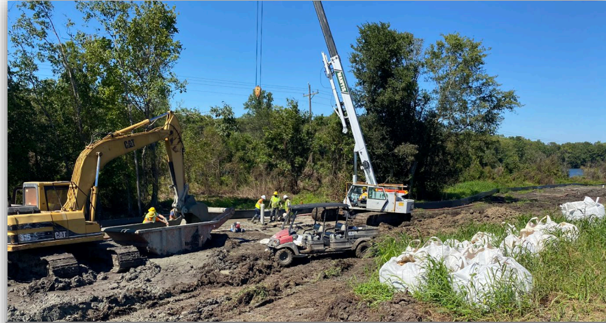
Well installation for Black Hawk Phase 2, Concordia Parish, October 2021
