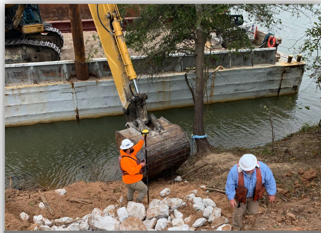
2016 Project, levee grade check
