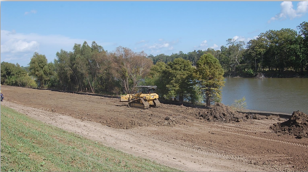
Placing levee embankment, MRL Item 401-R, Tensas Parish
