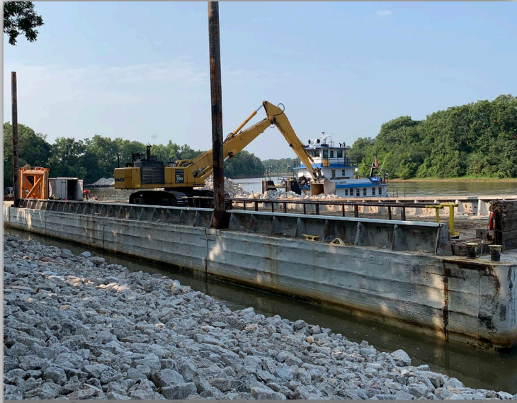
2016 Project, stone bank paving
