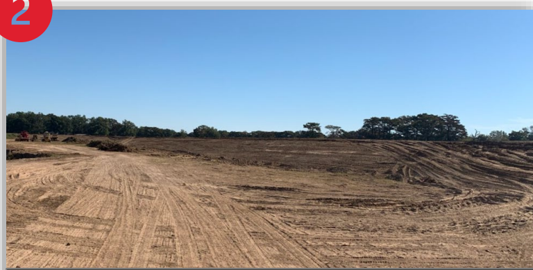
Finished levee, 2016 Project
