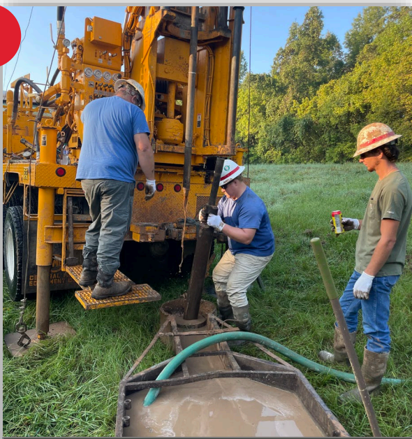
Borings being collected, 2019 Red Chute Project
