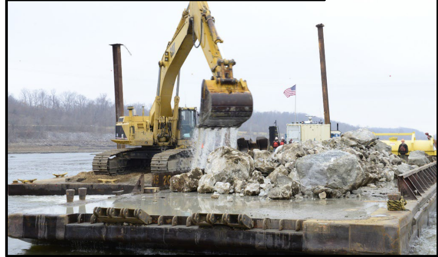
Rock Pinnacle removal at Thebes, IL
