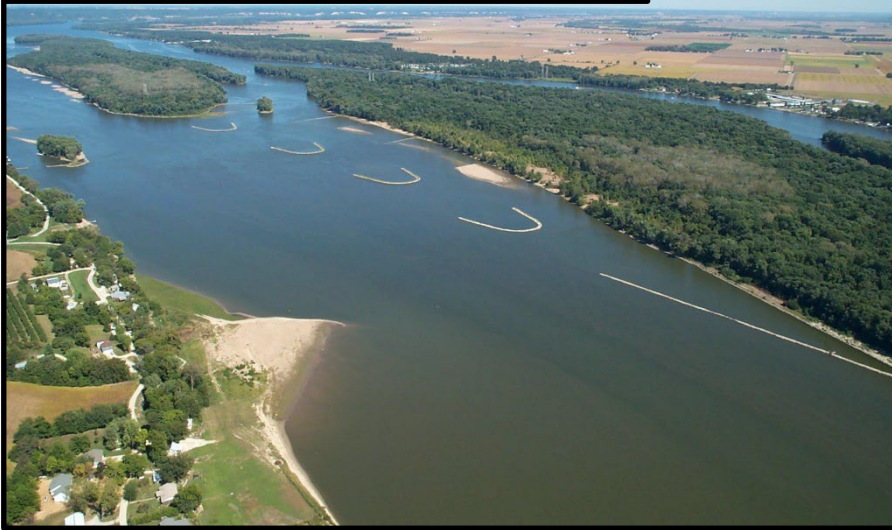
Aerial view of dikes on the MS River
