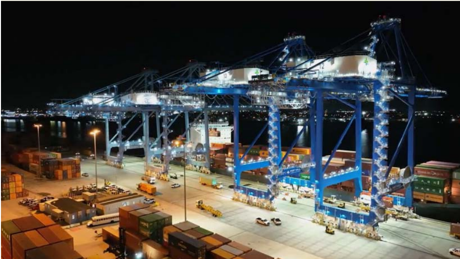
Port NOLA – Crane Rail Extension
