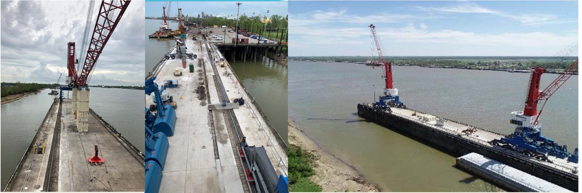
Port of South Louisiana – Harbor Cranes
