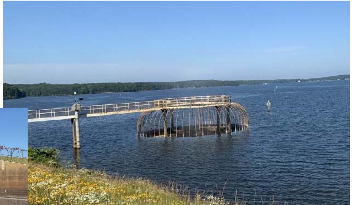
Morning Glory Inlet at Lake Claiborne Dam, Claiborne Parish
