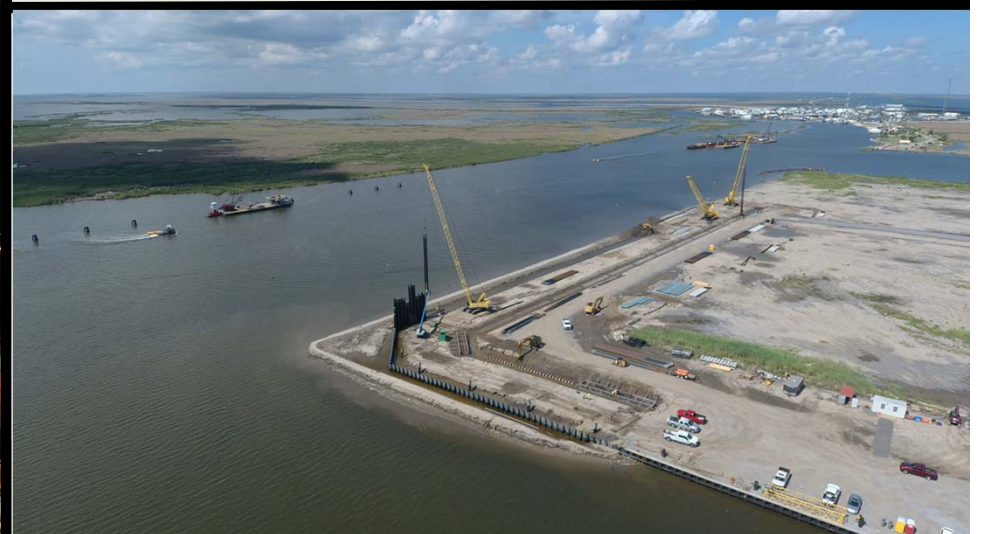
Port Fourchon – Bulkhead
