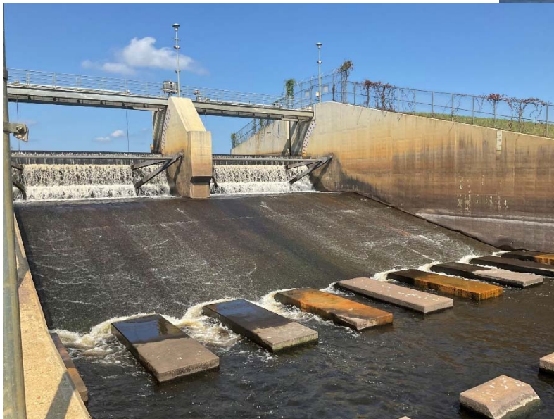
Tanter Gate Spillway at Bayou D'Arbonne, Union Parish
