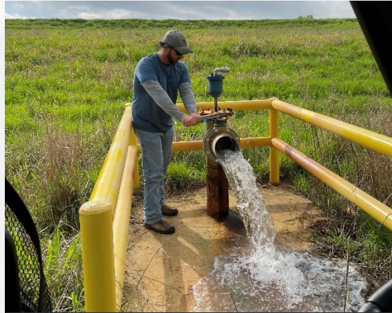
Testing the relief well valves at 329-R Blackhawk Phase 2, Concordia Parish
