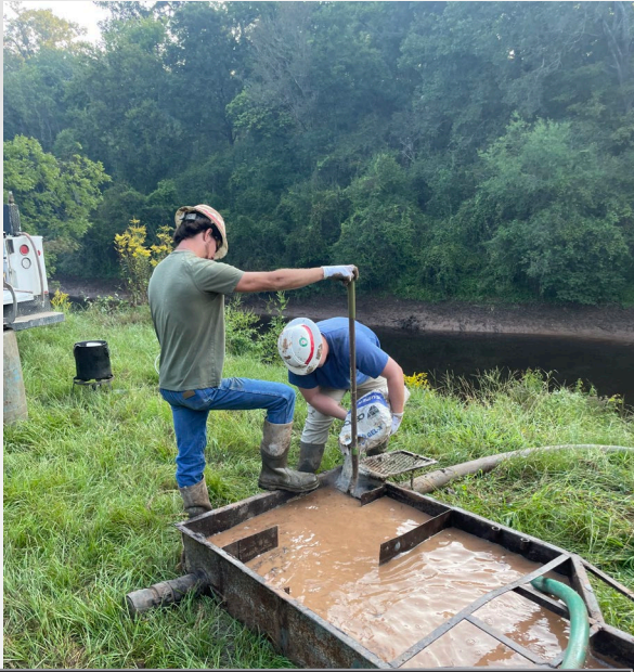
Borings being collected, 2019 Red Chute Project
