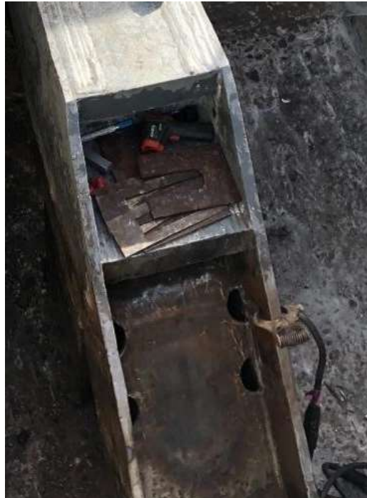
Boggs Miter Gate Repair
